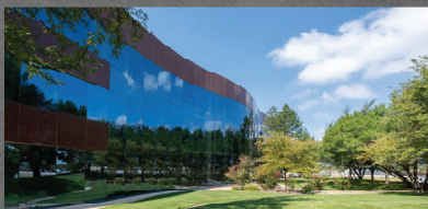
ZACHRY BUILDING 5601 I-40 West
