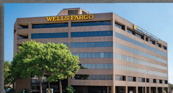
WELLS FARGO BUILDING 905 S Fillmore
