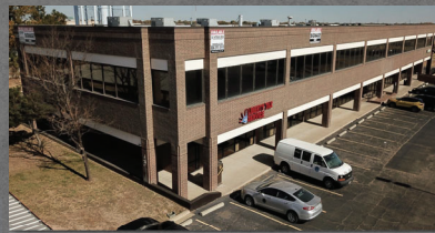
SOUTHTREE OFFICE PARK 5809 S Western
